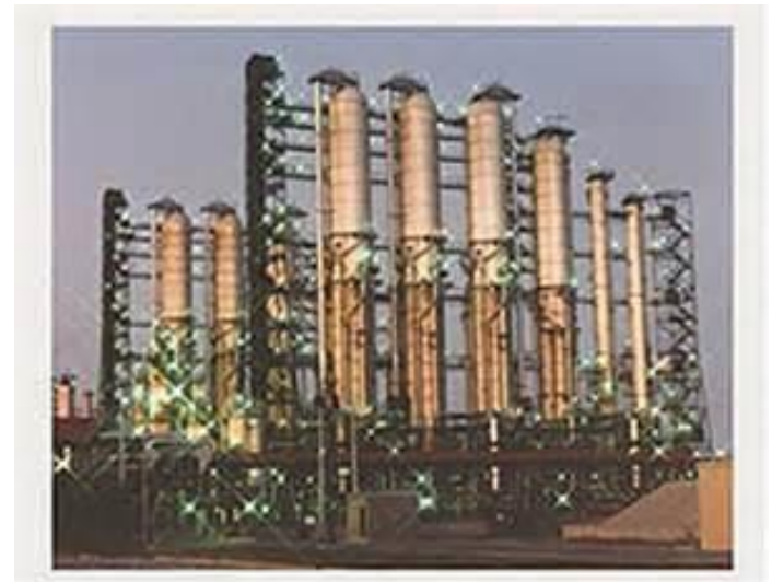
Bruce Heavy Water Plant
