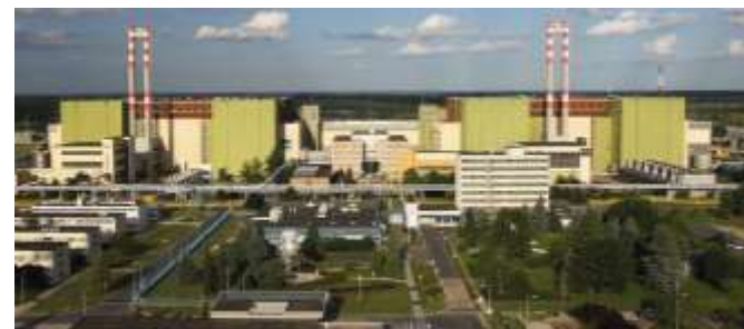
Paks Nuclear Power Station, Central Hungary
