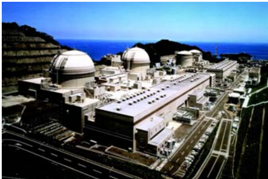
Ohi nuclear power plant, Japan (photo courtesy Kansai Electric Power Company).
