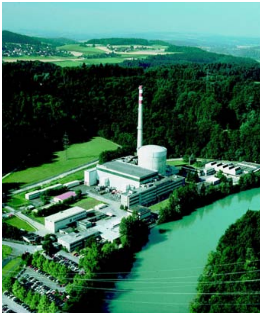
Mühleberg nuclear power plant, Switzerland (photo courtesy Bernese Power Utility).
