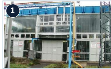
Hydrogen production building
