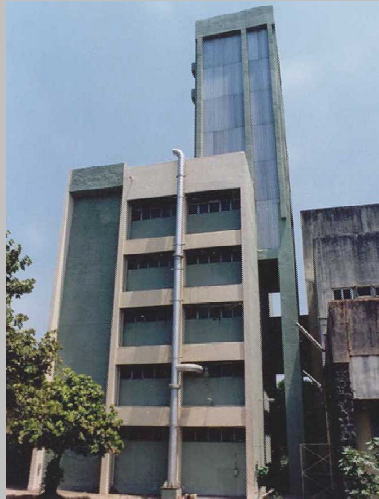
Integral Test Loop (ITL): A scaled test facility based on power to volume scaling for thermal hydraulic simulation of AHWRs
