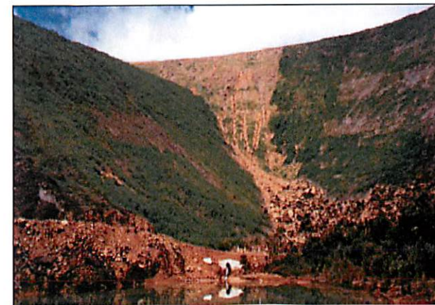
AFTER: Remediation completed
