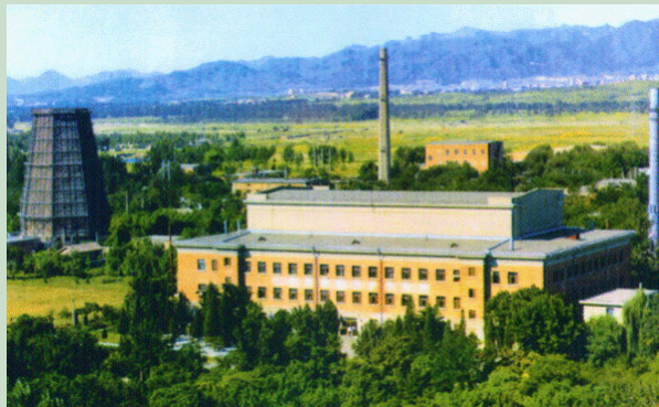
HWRR reactor building and cooling tower
