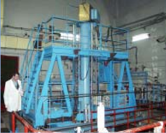
RMZ installation before dismantling
