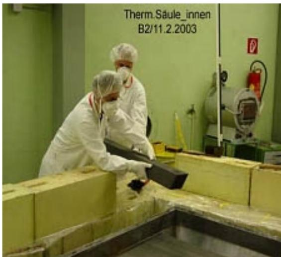
Figure 2. Inner thermal column – removing the graphite
