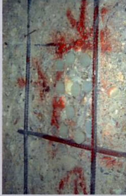
Figure 3: Drilling Field with Sealed Drilled Holes
