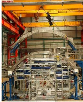
*Figure 5 : OIS installation onto a TF coil*
