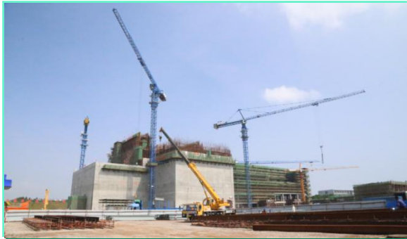
Civil Work of Nuclear Island
