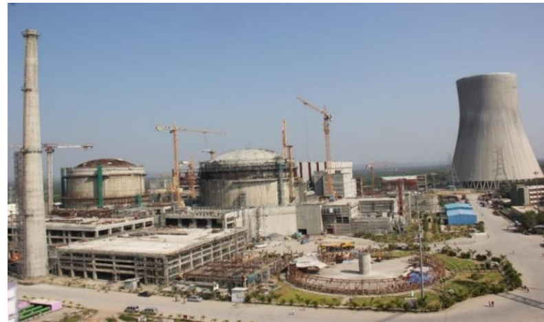
700 MW PHWR UNDER CONSTRUCTION
