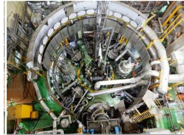
Reactor Assembly - PFBR
