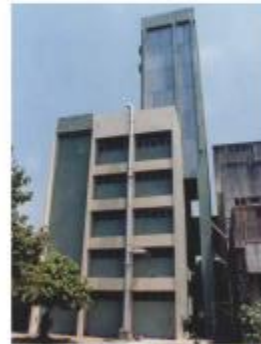
Building housing ITL
