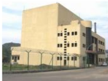
AHWR Critical Facility
