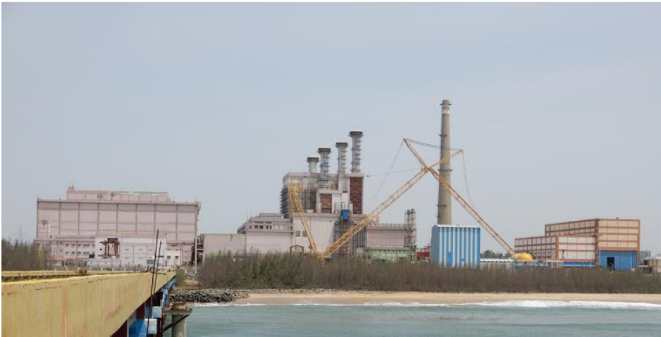
PFBRs under commissioning
