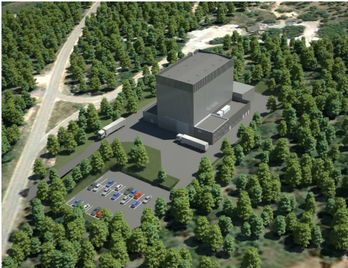
FIG. 1. Overall view of CHEOPS Facility
