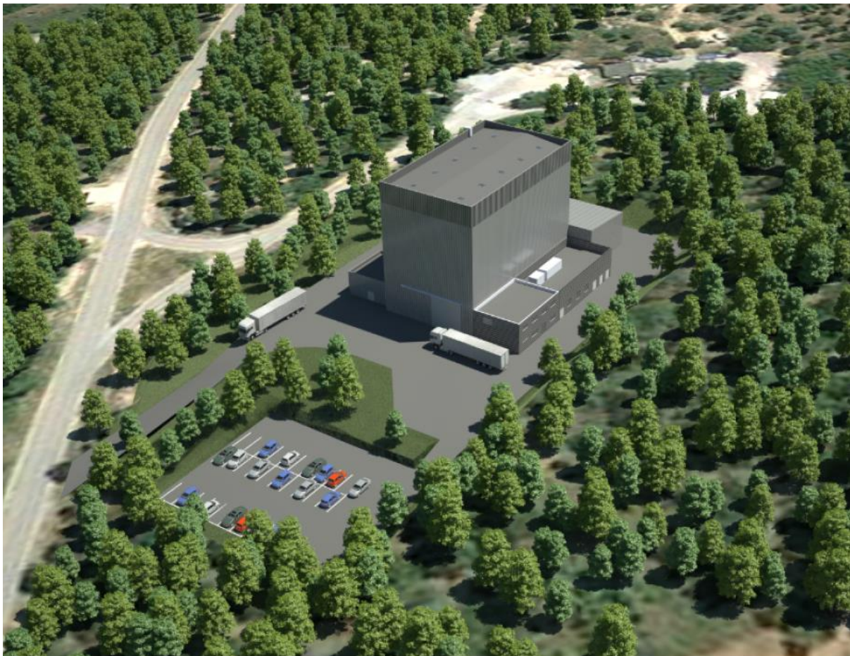
FIG. 1. Overall view of CHEOPS Facility
