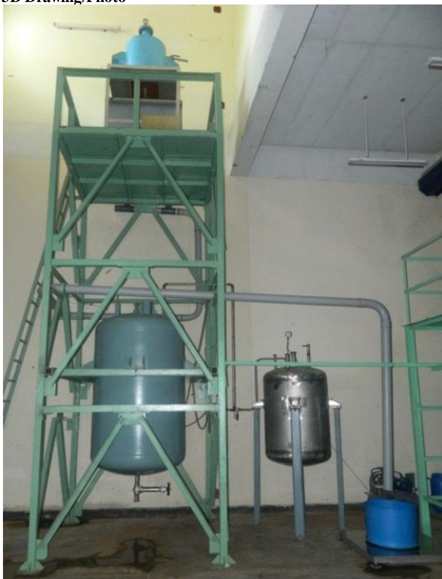
FIG. 2. View of the LCTMF mock-up facility
