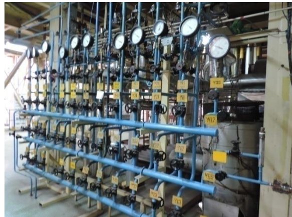
FIG.4. LCTR Cover Gas Header.
