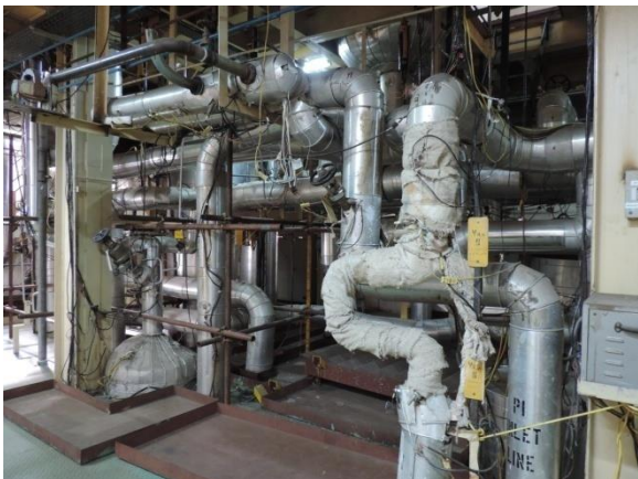
FIG.3. Purification Circuit and Sampler Unit.
