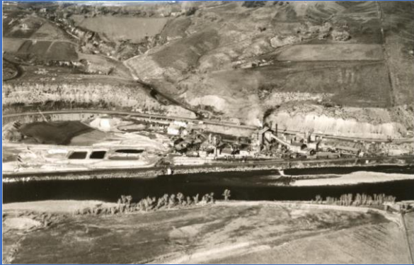
Rifle Mill tailings site
