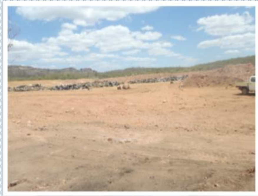
2013 – removal of the interim water management pond
