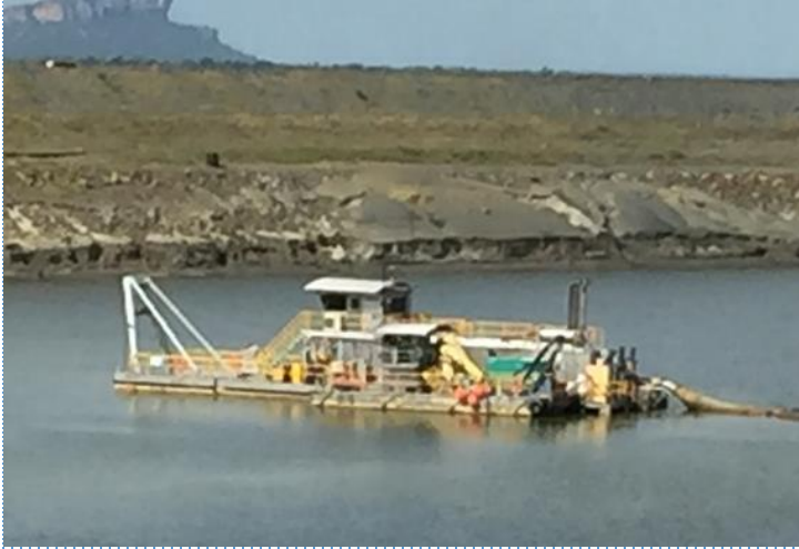
Dredge on Tailings dam - current
