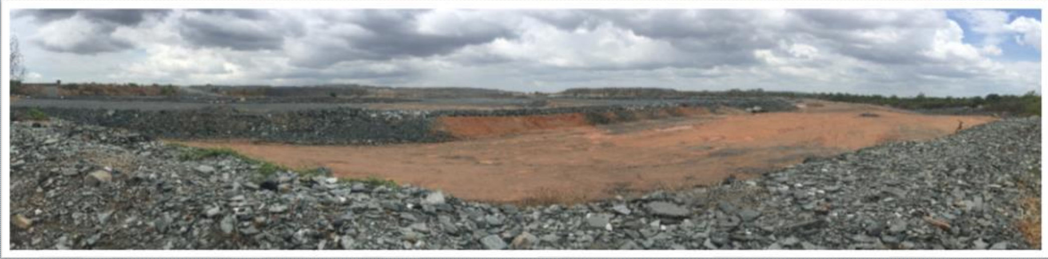
Pit 1 Backfill in progress
