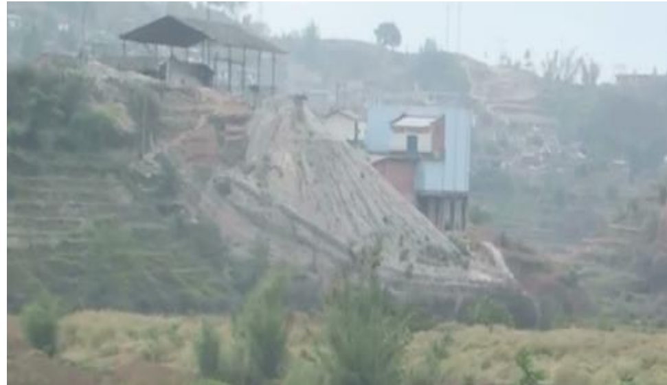
A waste storage
