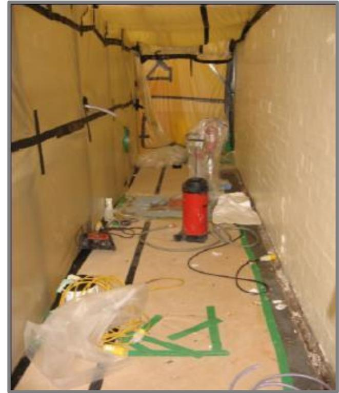
Decontamination operation carried out in a specially erected tent to ensure prevention of spread of contamination. Airborne contamination monitoring is task related.
